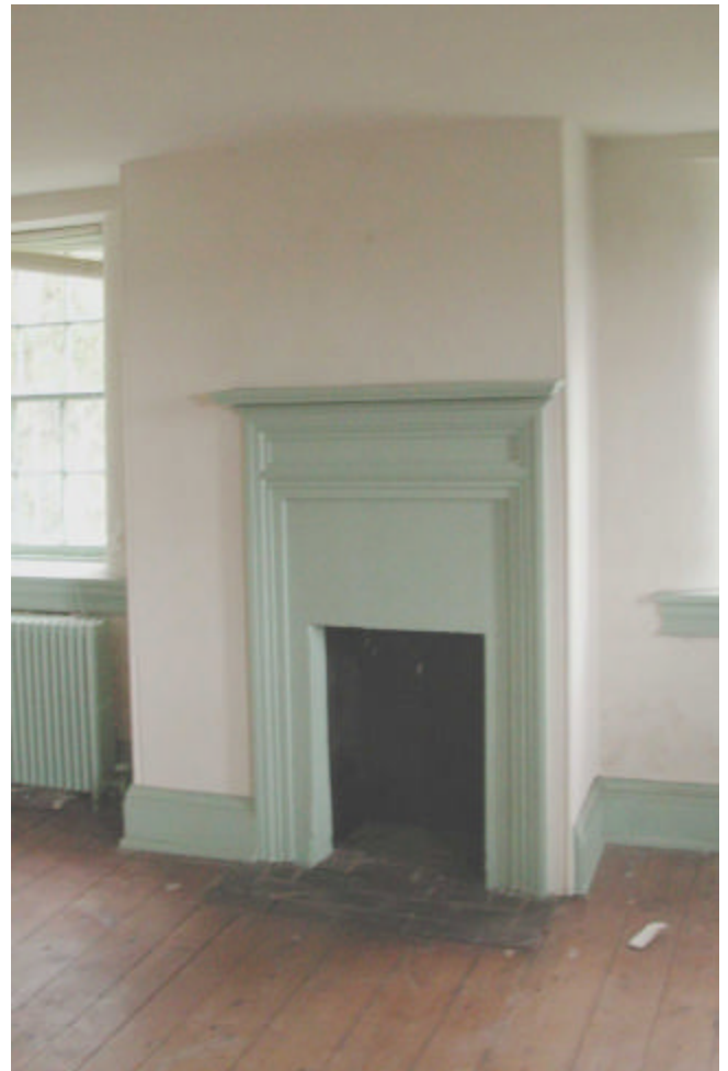
Second floor period IV fireplace, east end
