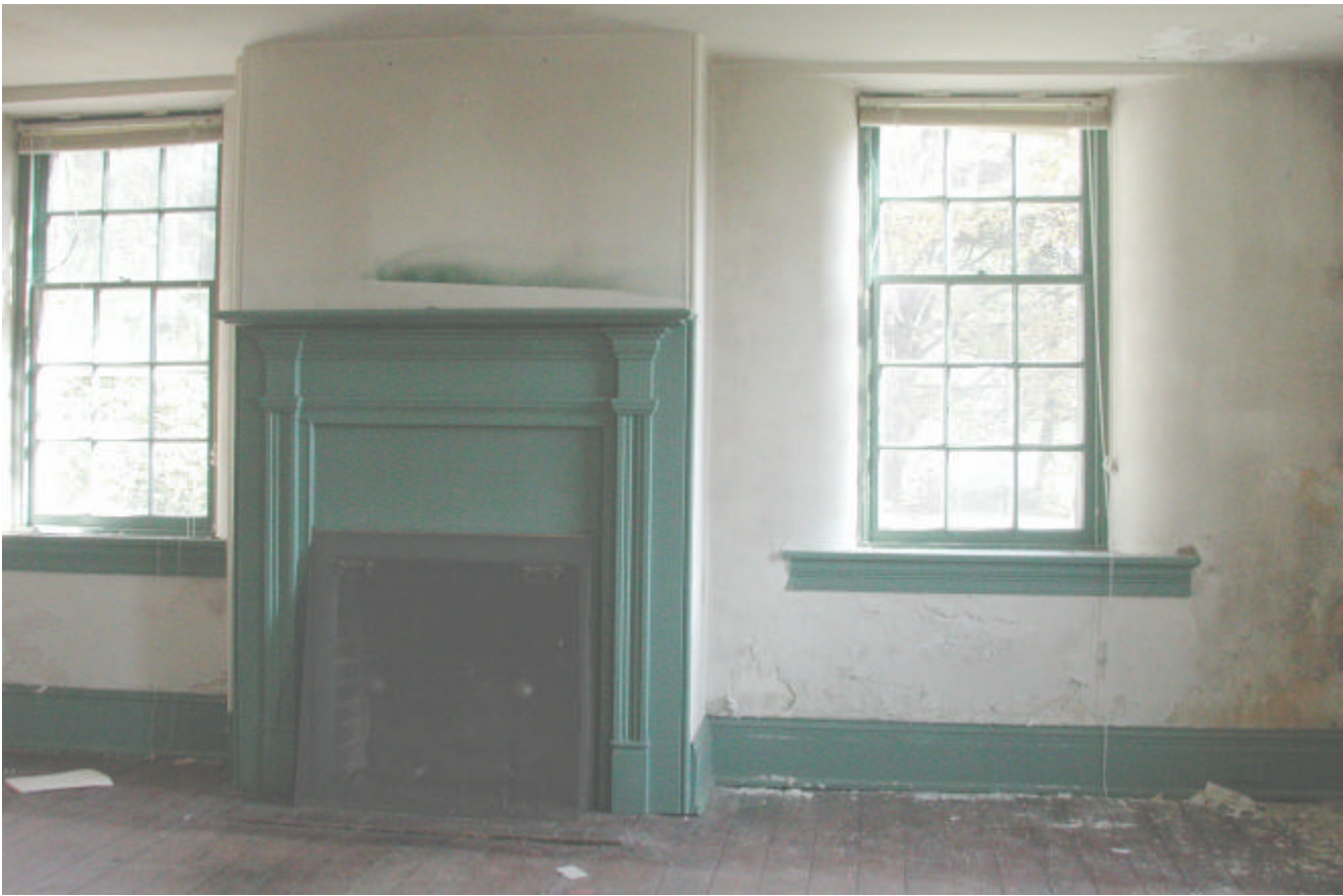
The period IV fireplace on the easternmost wall of the house, first floor. It was the most elaborate in the house and served the new period IV parlor.
